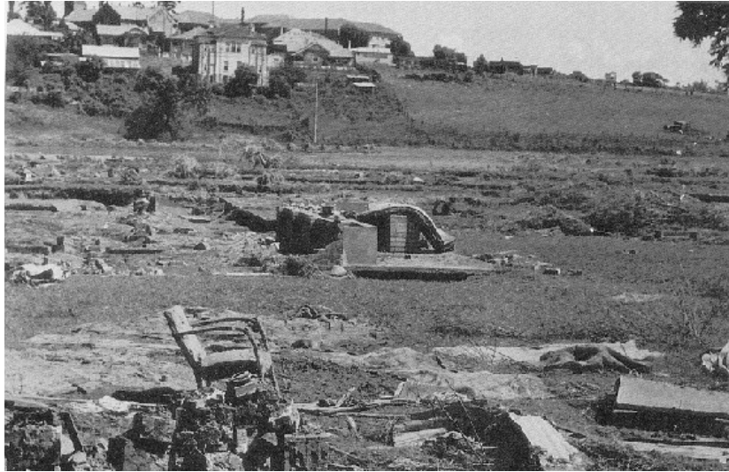
Before the flood a street of 20 houses stood there (Mount Pleasant Street, Maitland, 1995)
